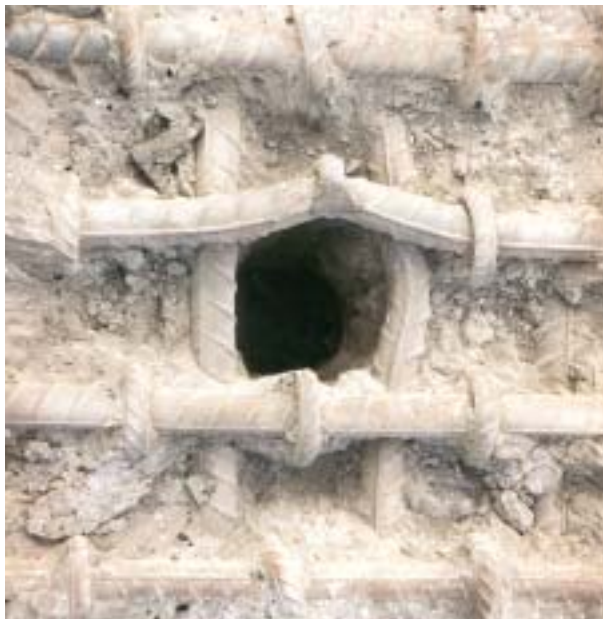
Figure 61. Post condition for reinforcement at back face of target 7 (shot 7).
