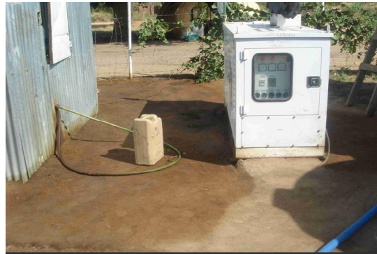
Fig 2. Oil pollution around generators – an everyday concern (photo S. Sundström FOI/the Swedish Armed Forces)
