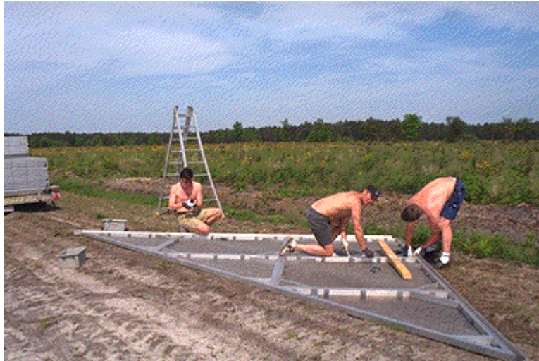
Figure 18. Deployment of FOA trihedral #1: The first triangular panel is mounted together from three square and three triangular sections. The short side length is 5.1 m.
