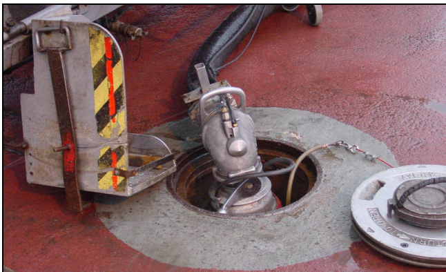
Figure 5-16. A pit where fuel is taken for refuelling. Photo by Michael Bracha, 2002, Linde Gas, Germany.
